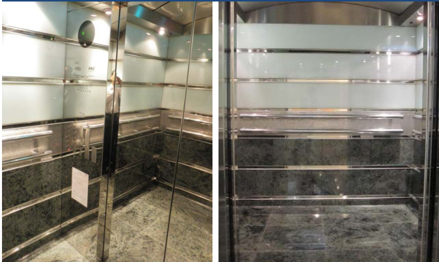
Prosperity Place Lift Renovation – Before
