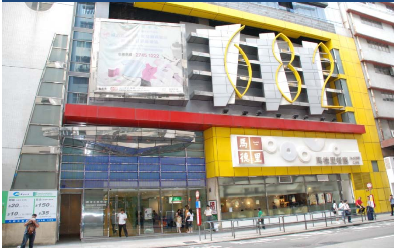
Trendy Centre Façade – Before
