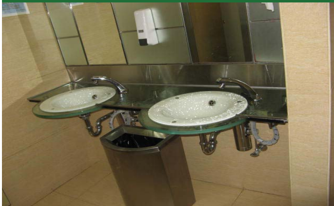
Metropolis Tower Washroom Upgrade: Before
